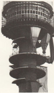
The first of the giant aerials is fitted into position.
